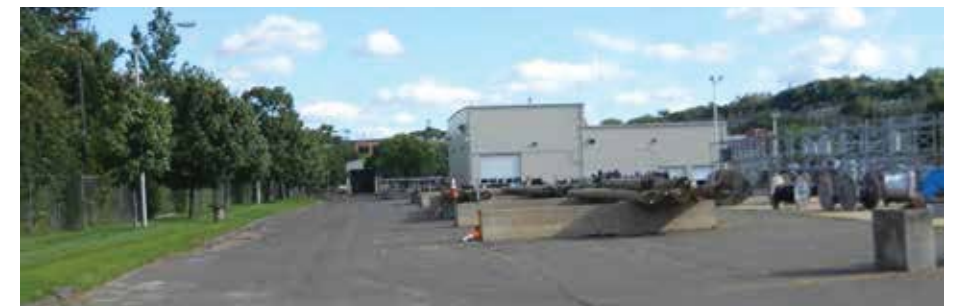
Existing conditions at the Connecticut Light & Power Co.
