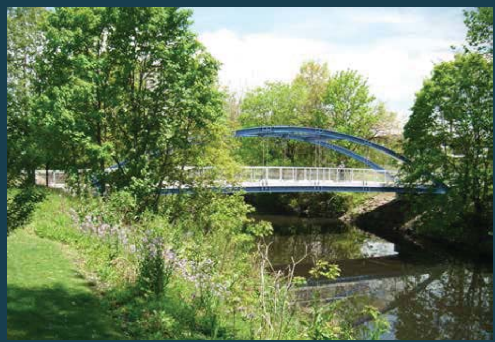
Example of pedestrian bridge over the Mad River
