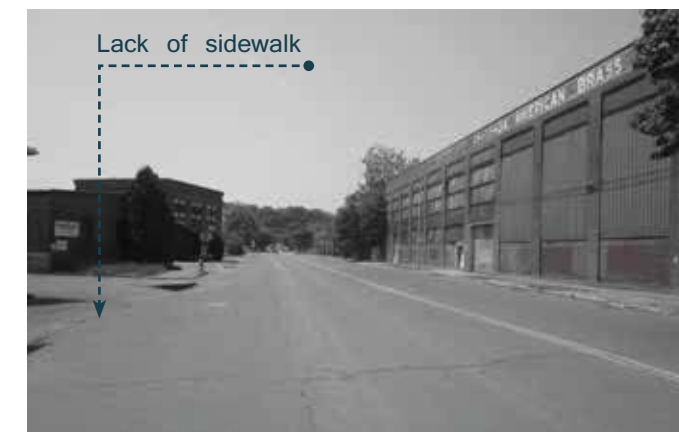
Existing conditions at Freight Street
